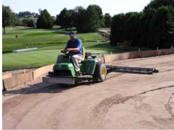
Dragging weighted ladder to float green.
