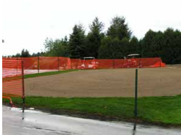
Fencing installation prior to fumigation process.
