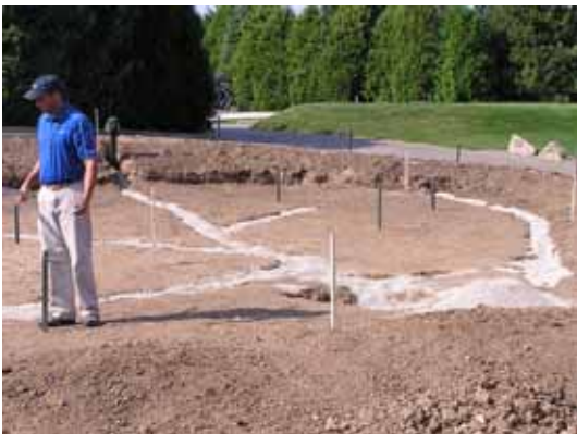
Herring bone style drainage pipe installed
