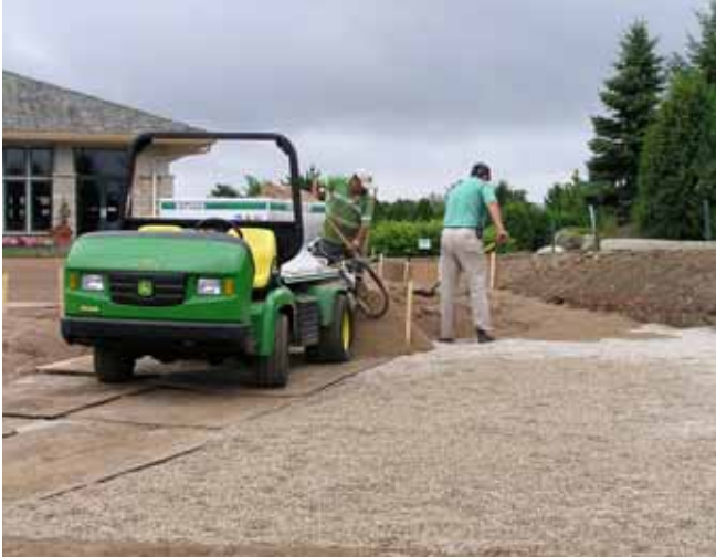
Plywood used to prevent crushing buried drain tile.
