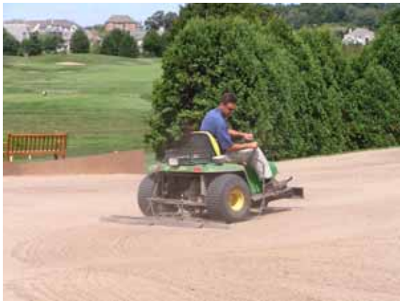
Raking in mix, blending existing and expanded areas.
