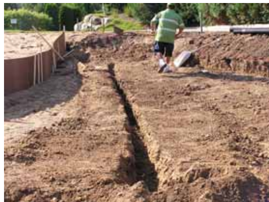
Trench prior to pipe and gravel bed install
