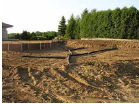
Laying out drain tile
