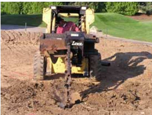
Trenching process for drain tile installation
