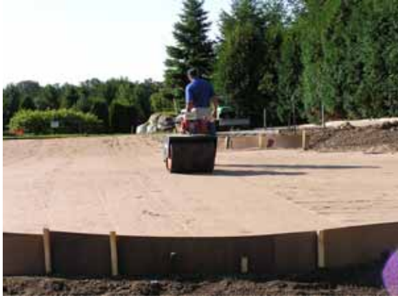
Rolling of greens mix, multiple directions for proper compaction
