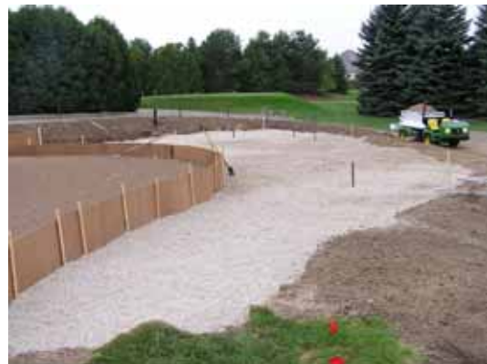
Four inch pea gravel layer installed.
