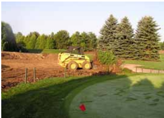
Removal of trees and start of cavity excavation.
